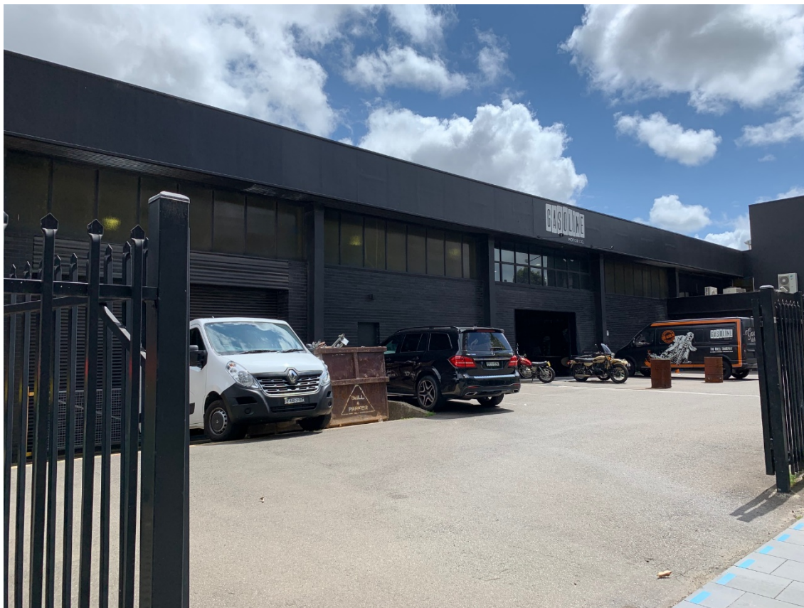
hardstand adjacent to east at 1037-1047 Bourke St
