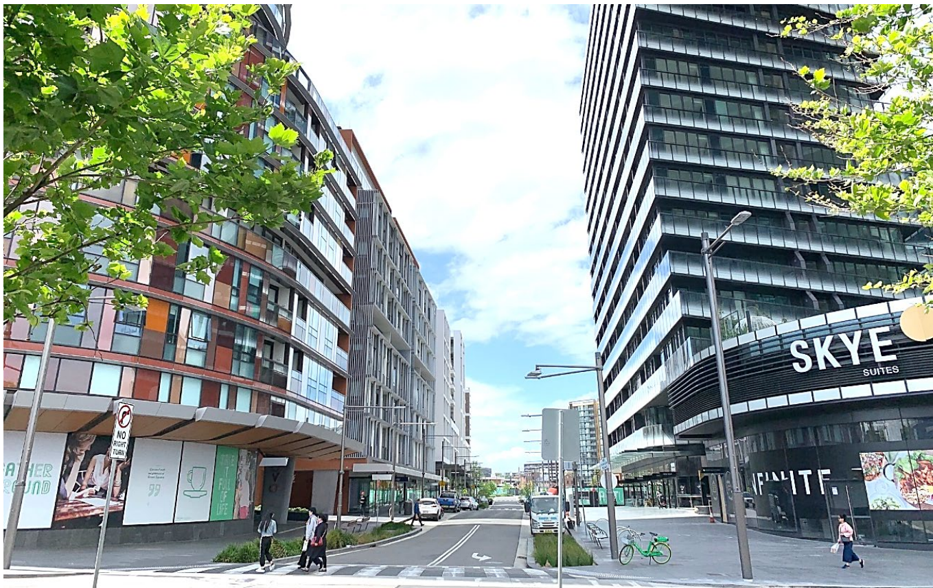
view south along Ebsworth Street from site
