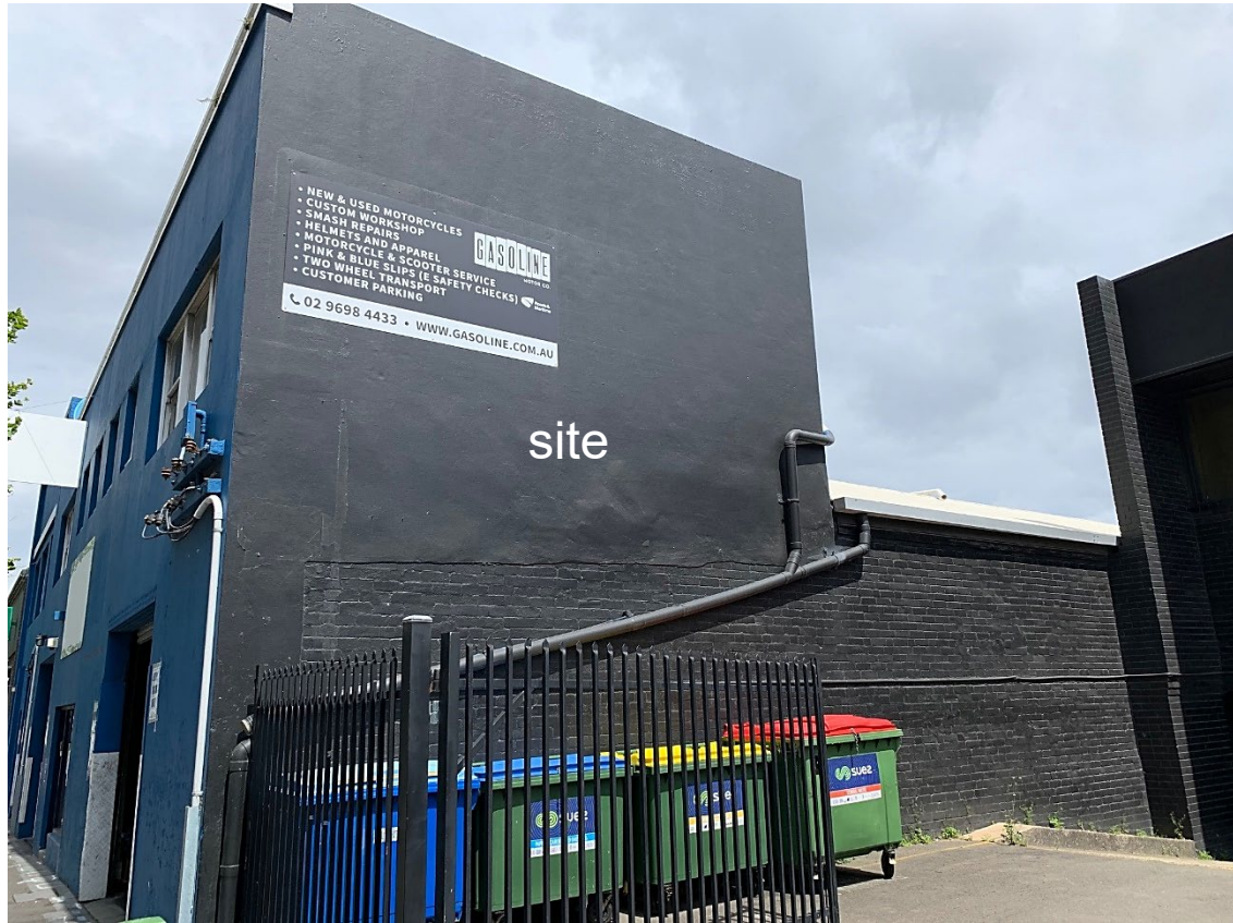
north-east elevation of existing warehouse building
